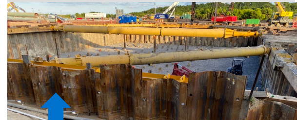
Sheet Piles (shoring of sandy soil)
